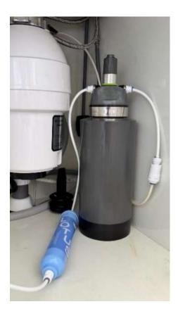
15. Screw gently the 3/4" connector into the Air-Release valve, ensure there is internal gasket. Do not use any tools.
