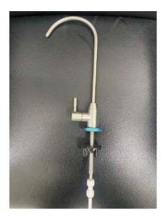
8. Tighten the faucet securely under the sink and attach the push-to-connect fitting to the threaded end of the faucet.
