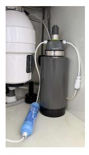
11. Screw the 3/4" connector into the Air-Release valve, ensure there is internal gasket.
